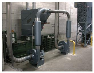
Sound attenuation devices at the infeed and inline cutter of 25 different presses keep this facility running smoothly and quietly for Diversified Labeling Solutions, Itasca, III.
