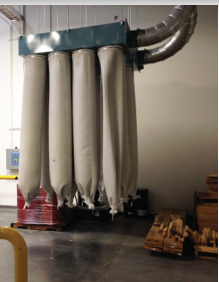
Filter plenum dust collector system for light duty applications where line down-time, hygiene and safety are secondary
